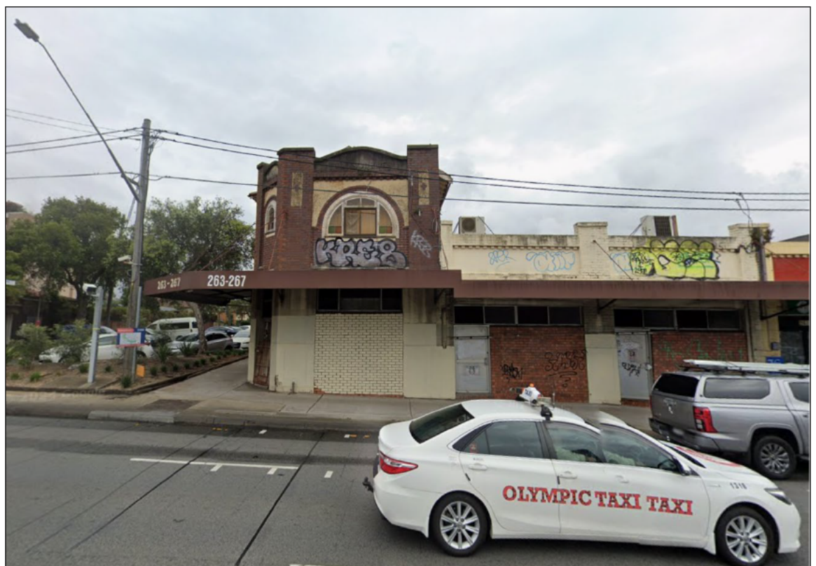
Figure 3: The site, as viewed from Canterbury Road (Source: Google).
